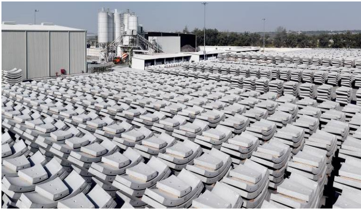
Up to 700 m 3 of concrete installed per day: Segment production plant for STEP in Abu Dhabi.
